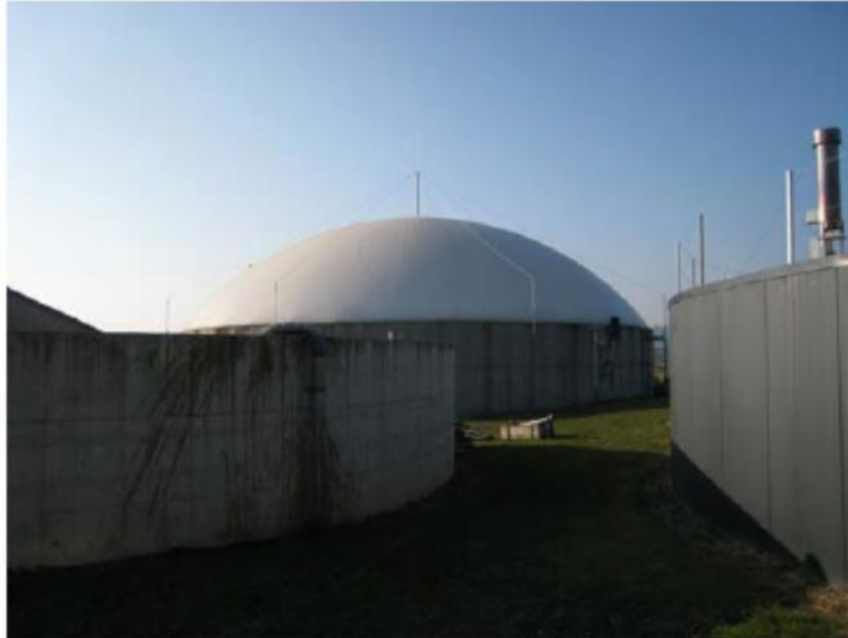
Figure 9: Biogas plant/fermentation tank with foil gas storage
