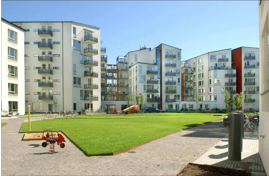
Picture 1: waste inlets installed in a court yard of a housing bloc in Hammarby Sjöstad.
