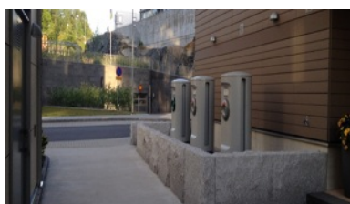
Underground waste collection system in the Gothenburg region, Sweden.
